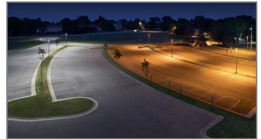
Installation of LED parking lot lights (left) compared with HPS lights (right) shows the difference in color and distribution.
